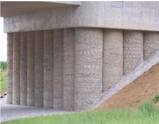
FIGURE E.1: Examples for piles with grooves, not affecting the minimum cover for durability
